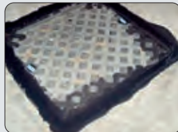
Scellage des cockpits
